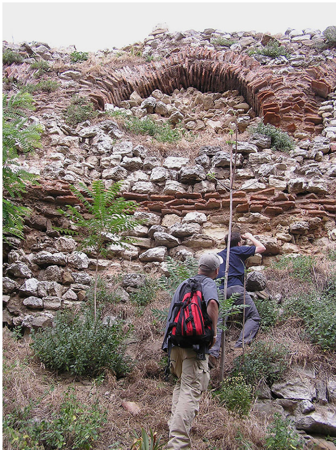
Fig. 10 — Brick blind arcade at the west walls at Silivri (© The author).
